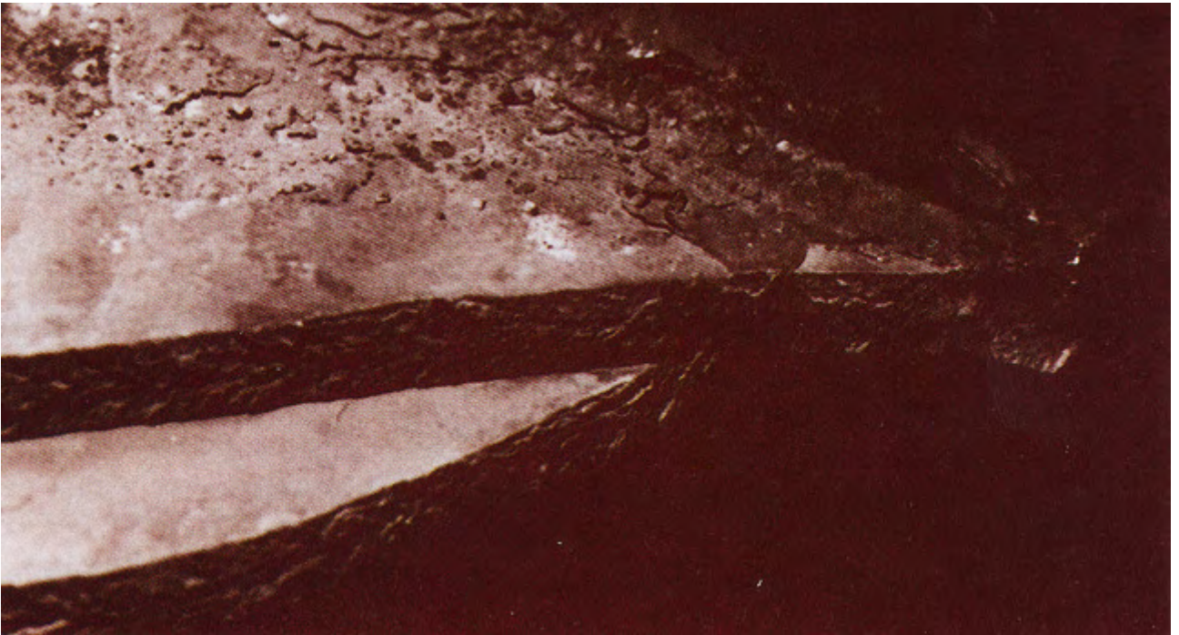
Fig. 4 Brittle fracture from manway to foot of tank (to the left).
