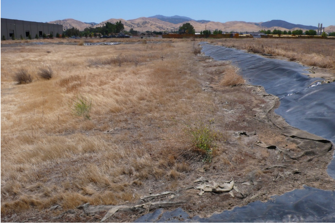
Photo 5. Northwest corner of detention basin looking south
