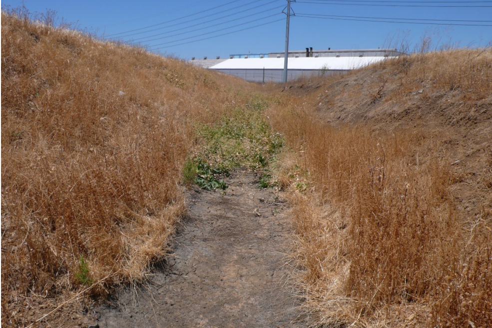
Photo 3. Bottom of drainage ditch
