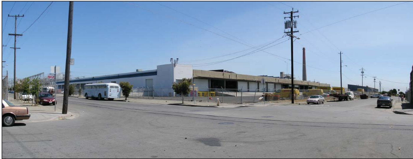
A Baseline view as seen from KOP SF-5 toward HWC (Mitigated) converter station site
