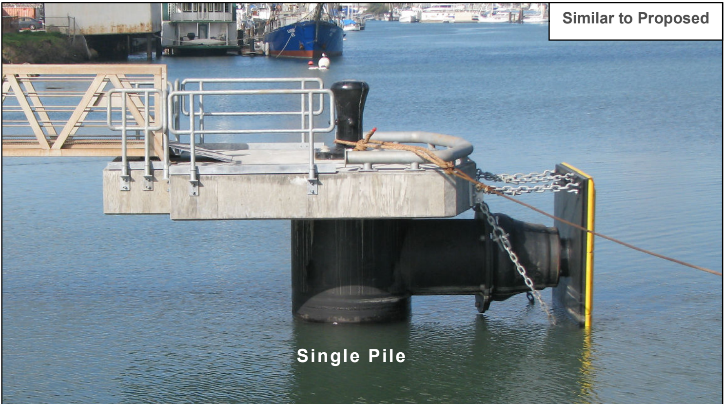
Figure 2-14 Existing and Proposed Breasting Dolphin City of Pittsburg WesPac Pittsburg Energy Infrastructure Project
