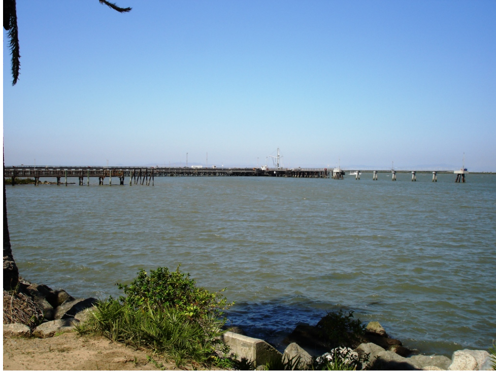
Photo 3-1: View of marine terminal from Riverview Park looking west
