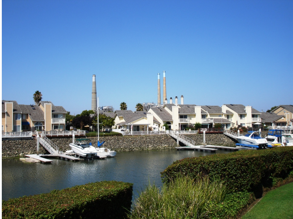
Photo 3-5: View toward storage terminal from residential area looking west
