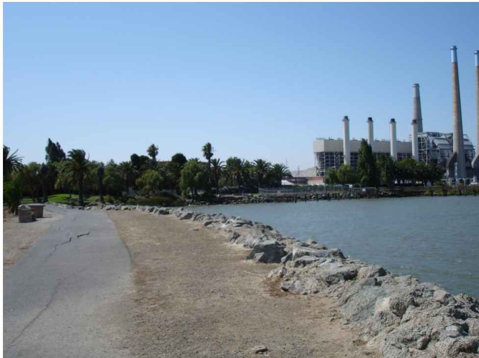
Photo 3-2: View of storage terminal from Riverview Park looking southwest
