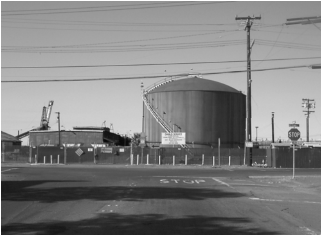
Ultramar Inc., a petroleum refining company located at Harbor Street and East Third Street, is one of Pittsburg's many industries.
