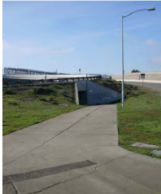
Pedestrian Tunnel under SR 4
