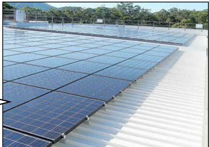
Solar Panels with Cool Roof Below
