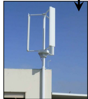
Low-Profile Roof Top Wind Turbines
