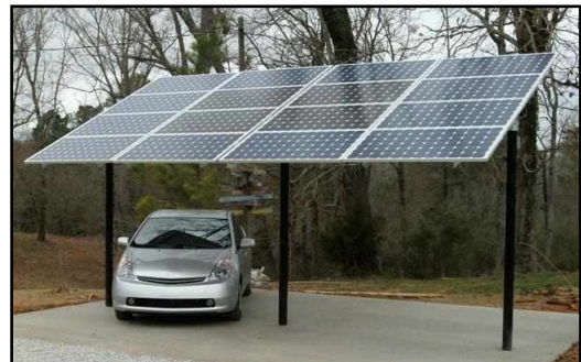
Solar Carport Example
