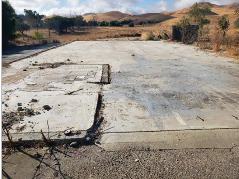
Figure 4. Overview of the Project Area (view south; September 26, 2023).
