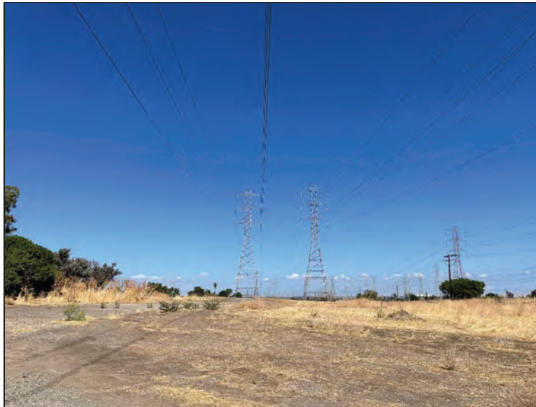
Figure 7. Overview of the Transmission Lines (view north; September 26, 2023).
