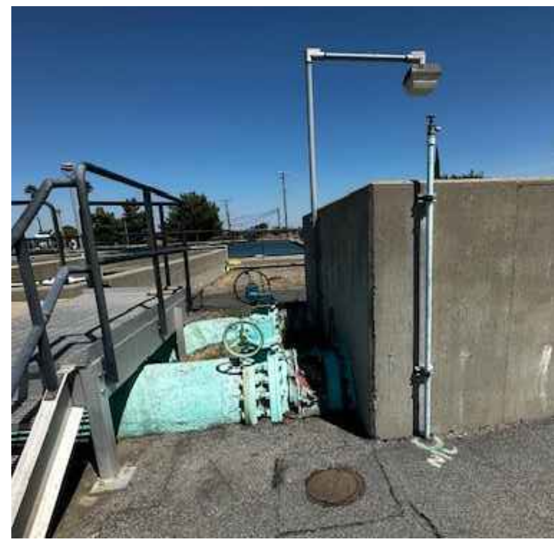
PICTURE 1 EXISTING 24" BFV'S (VIEW FROM EAST)
