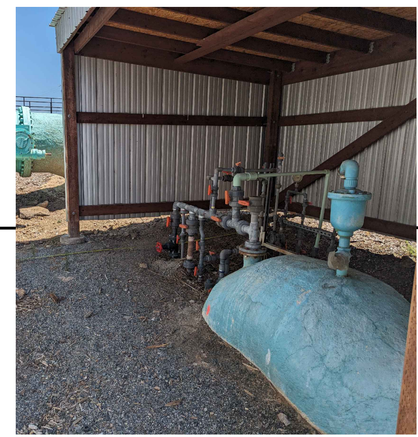
EXISTING INJECTOR BUILDING PHOTO 1
