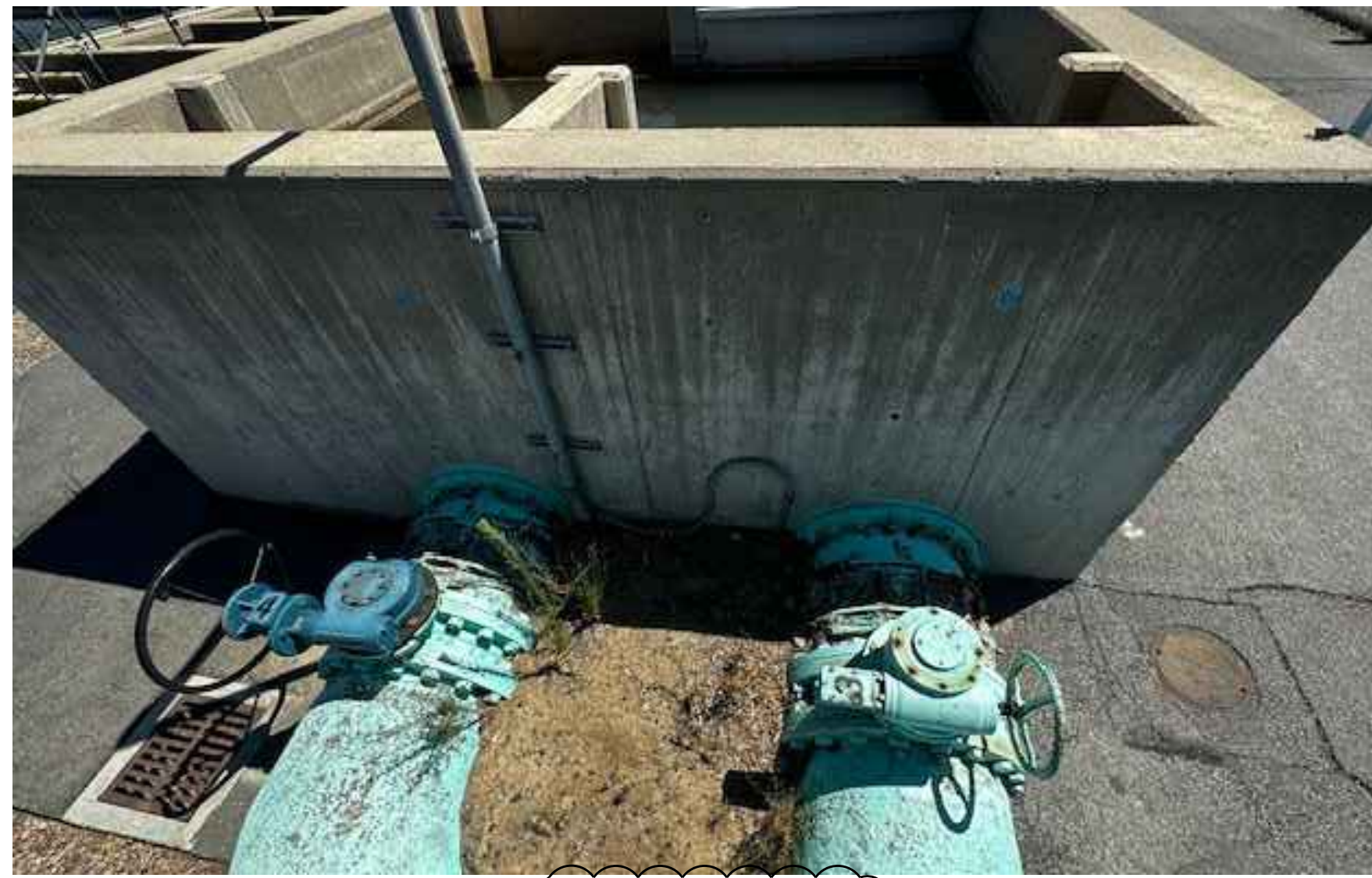
PICTURE 2 EXISTING 24" BFV'S (VIEW FROM TOP)
