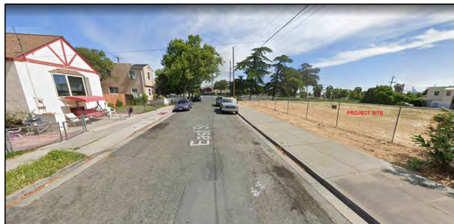
⑥ SITE VIEW FROM EAST STREET LOOKING NORTH
