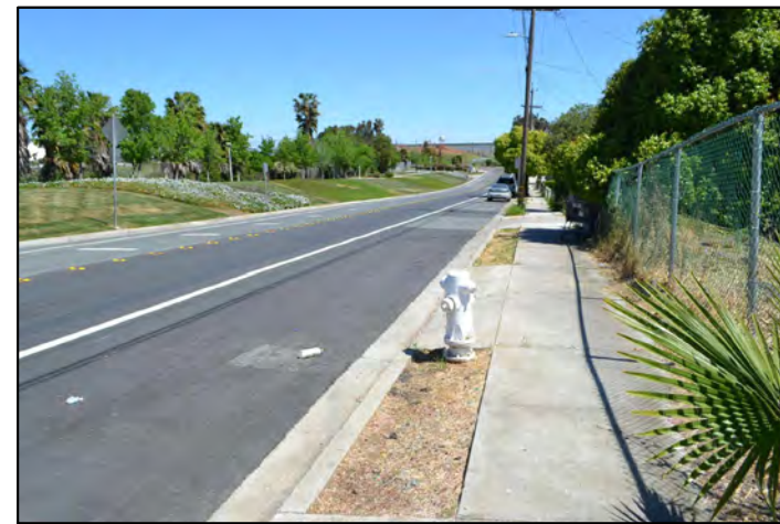
④ SITE VIEW FROM E. 8TH STREET LOOKING EAST
