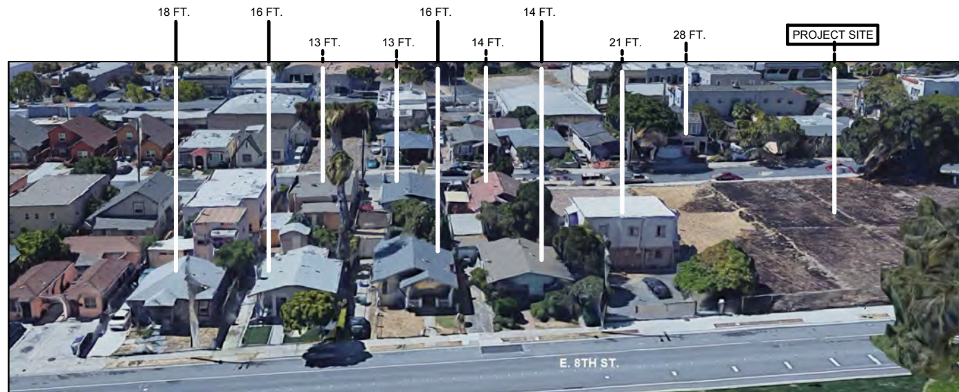
1 APPROXIMATE VICINITY STRUCTURES HEIGHTS - VIEW LOOKING SOUTH FROM E. 8TH STREET SCALE: NOT TO SCALE
