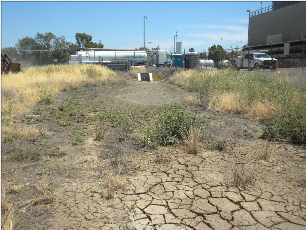
Photo 10: Sediment basin (lacks hydrophytic vegetation and soils) in southeast corner, facing east.
