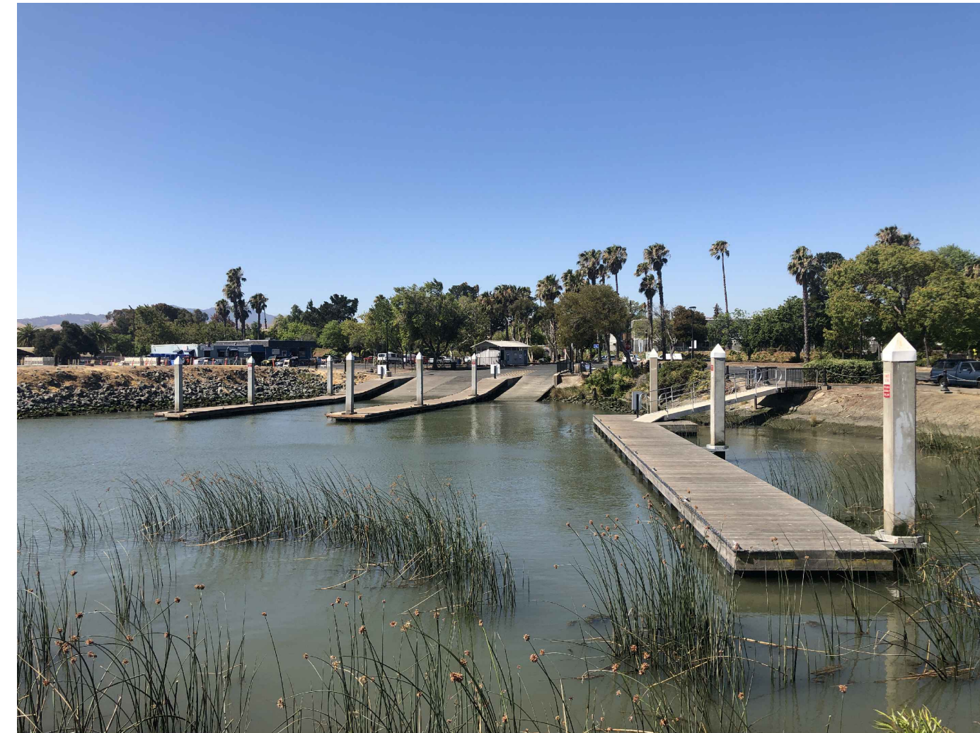
PHOTOGRAPH 4 LAUNCH AREA FLOATING LAUNCH DOCKS (DREDGE AREA B)
