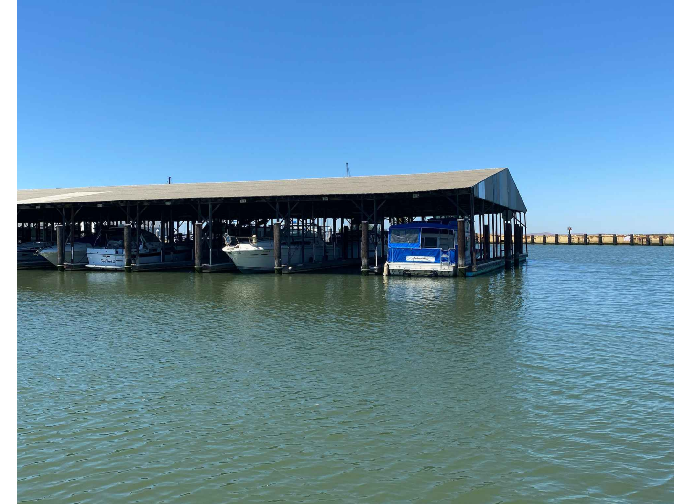
PHOTOGRAPH 3 BASIN 3 DOCK COVERS (DREDGE AREA A)
