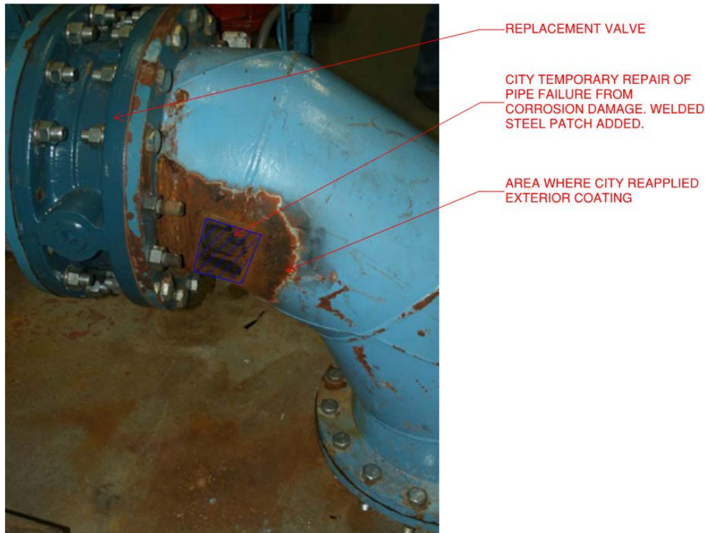
Figure 1-1. Repaired Filter 7 Backwash Inlet Elbow
