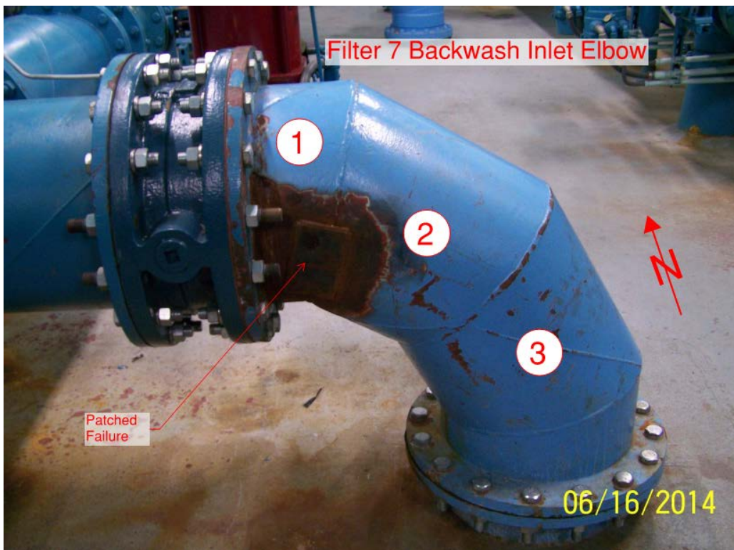
Figure 2-1. Filter 7 Backwash Inlet Elbow Measurement Locations
