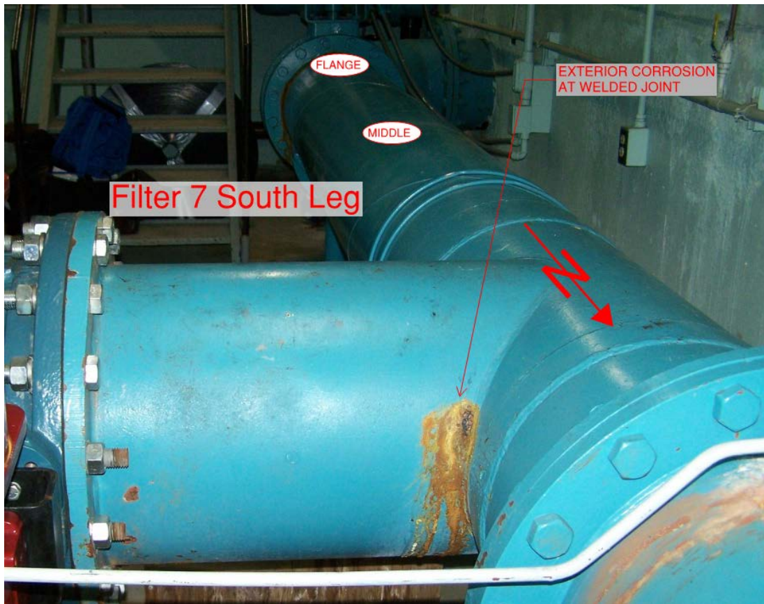
Figure 2-3. Filter 7 South Leg Measurement Locations
