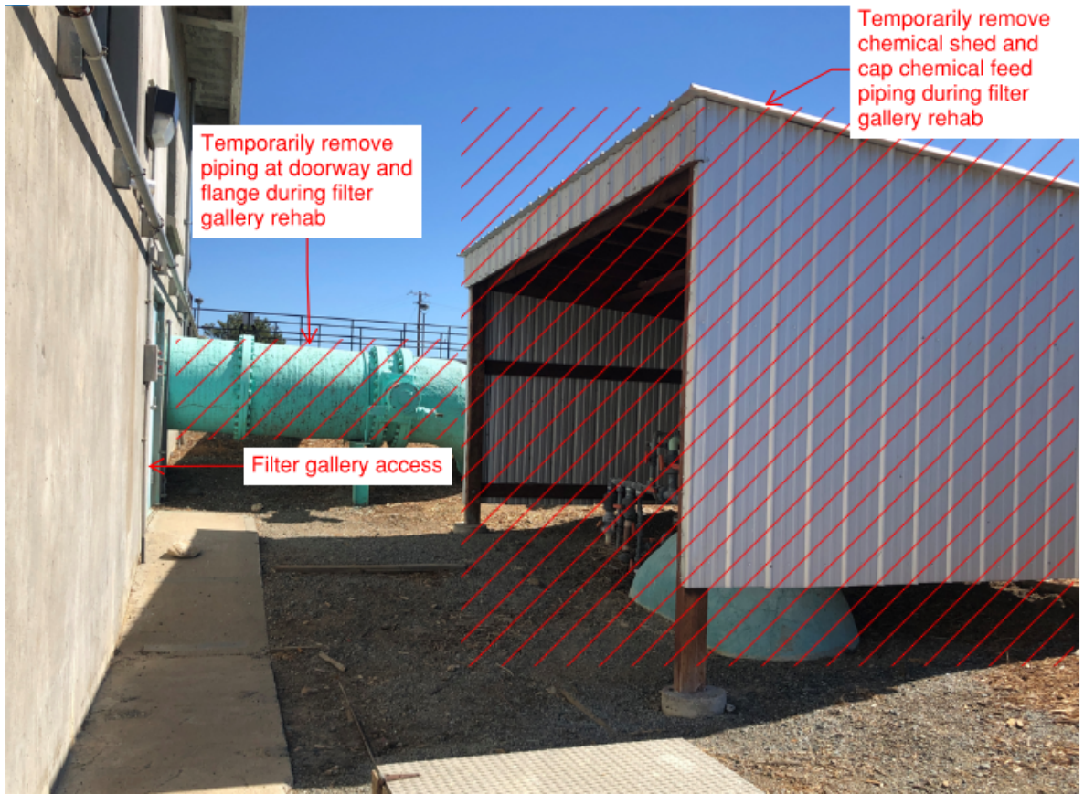
Figure 2-6. Temporary demolition needed for access to filter gallery during construction
