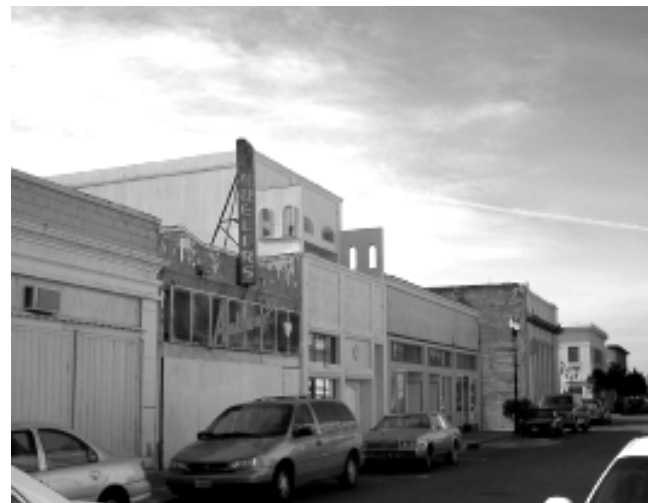
The south side of East Fourth Street demonstrates the City’s unique historical character.
