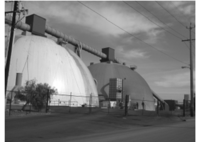
Sites such as the storage site of petroleum coke dust for Koch Carbon, located on East Third Street could provide redevelopment opportunities for the City.
