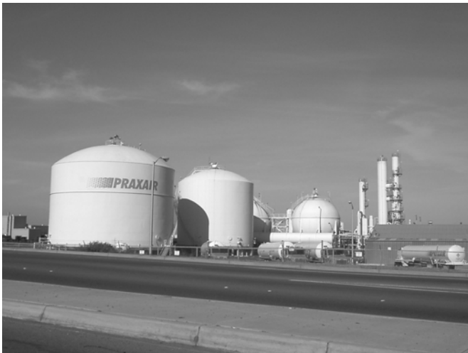
Praxair facility located on California Avenue at Loveridge Road intersection supplies atmospheric, process and specialty gases, high-performance coatings, and related services and technologies.
