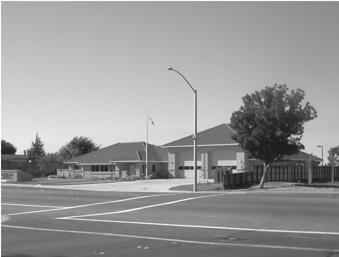
Fire Station #87 on West Leland Road serves both Pittsburg and Bay Point residents.
