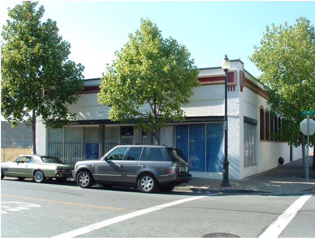
Photograph 1. Scampini Building NW Elevation
