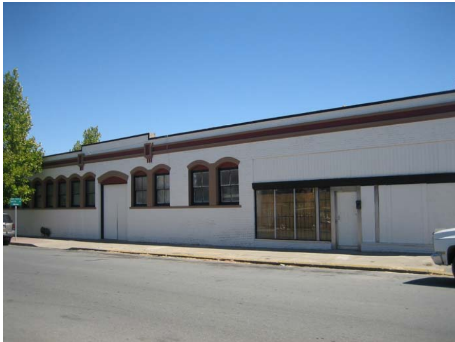
Photograph 2. Scampini Building, West Elevation
