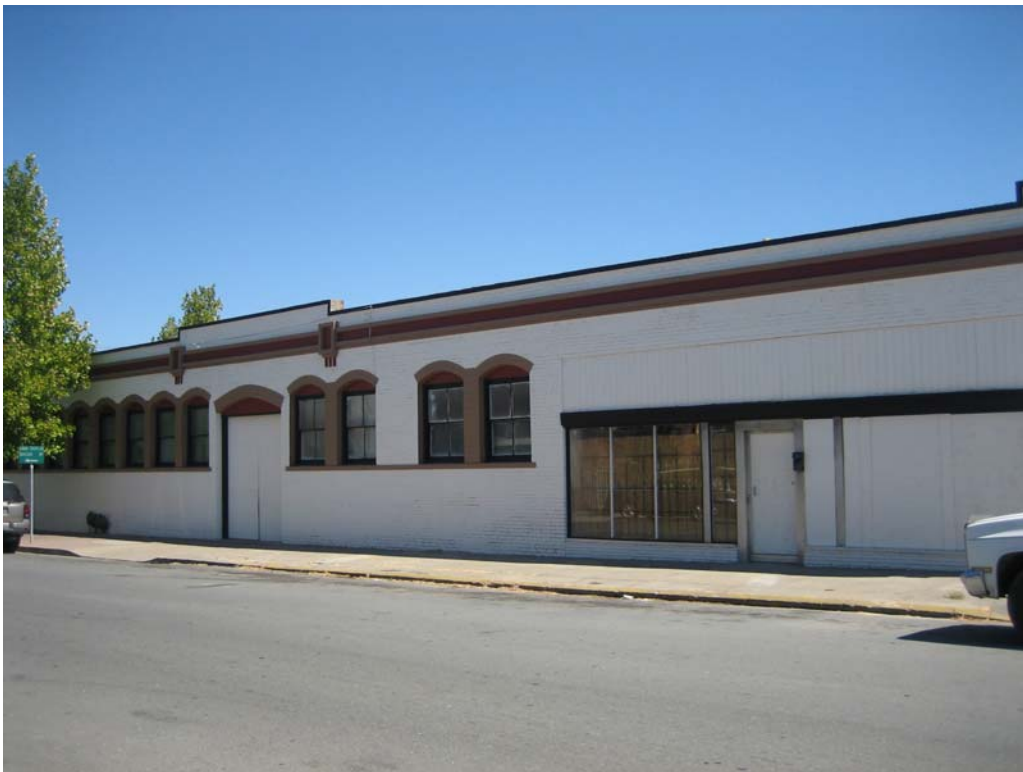
Photograph 2. Scampini Building, West Elevation
