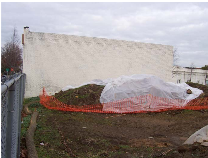
Photograph 3: Scampini Building, South Elevation
