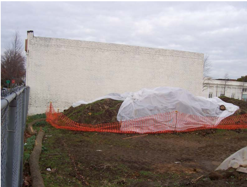
Photograph 4. Scampini Building, South Elevation
