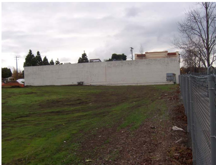
Photograph 4: Scampini Building, East Elevation
