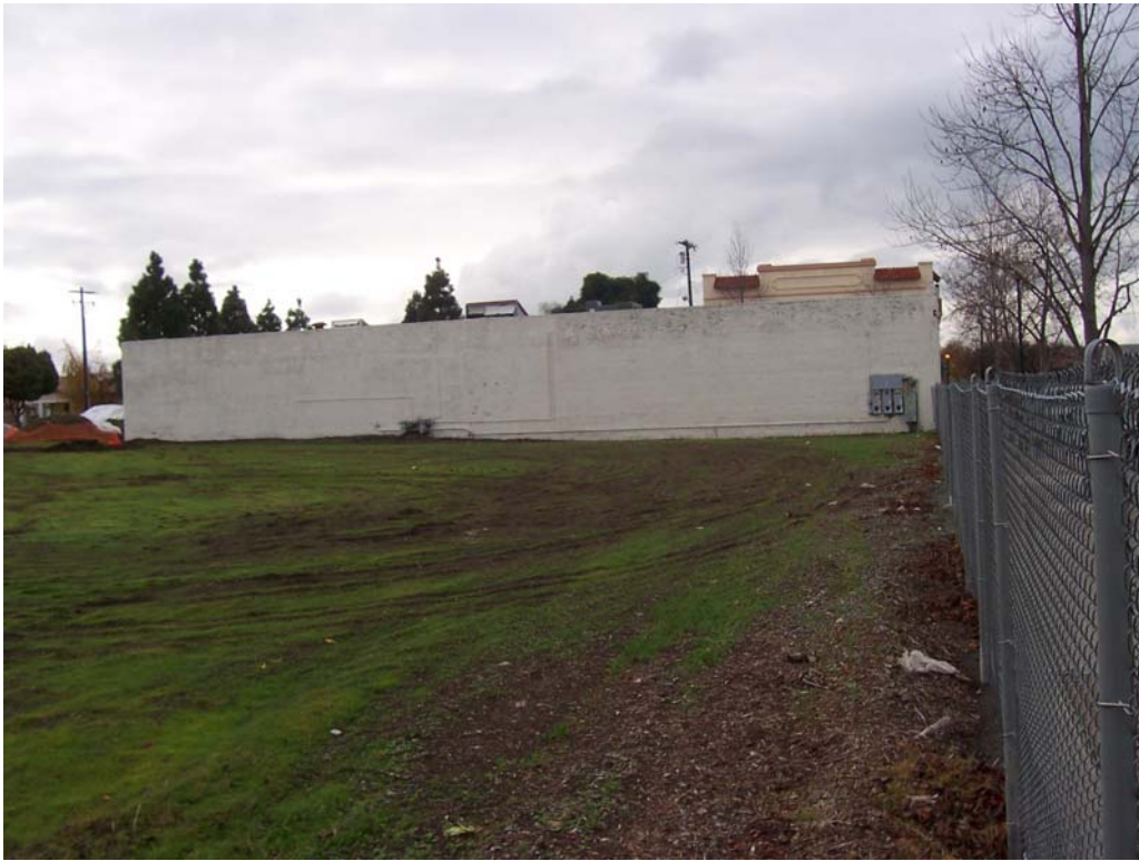
Photograph 3. Scampini Building, East Elevation
