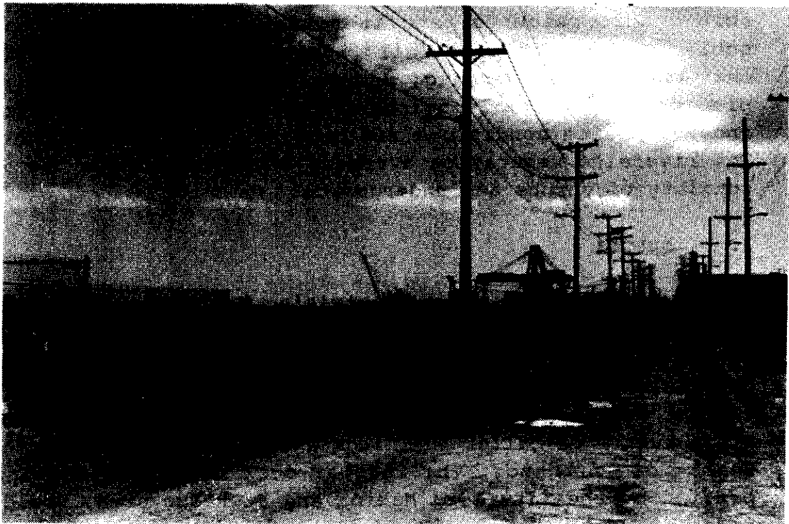
Figure 41 SITE PHOTOGRAPH: PRIVATE EXTENSION OF EAST THIRD STREET Han-Li International Marine Terminal EIR City of Pittsburg, California
