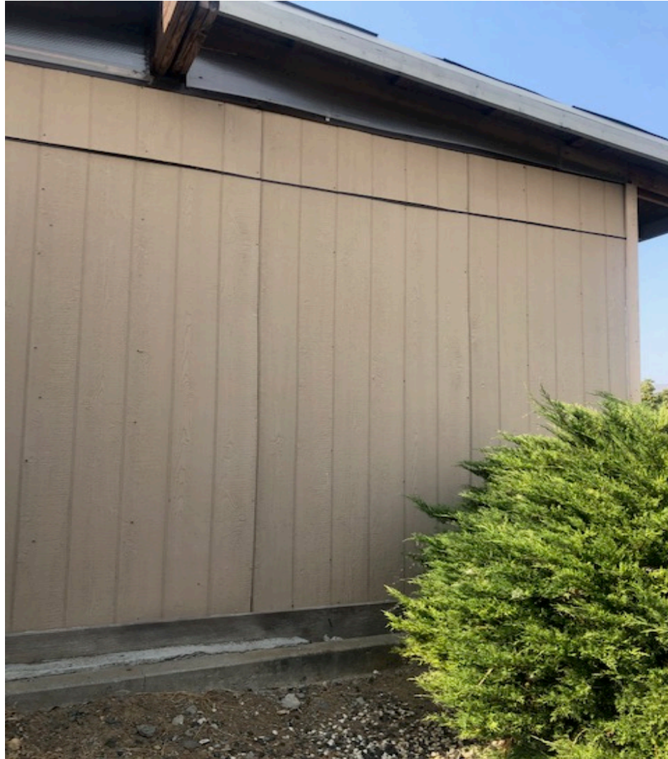
View of structure from the east
