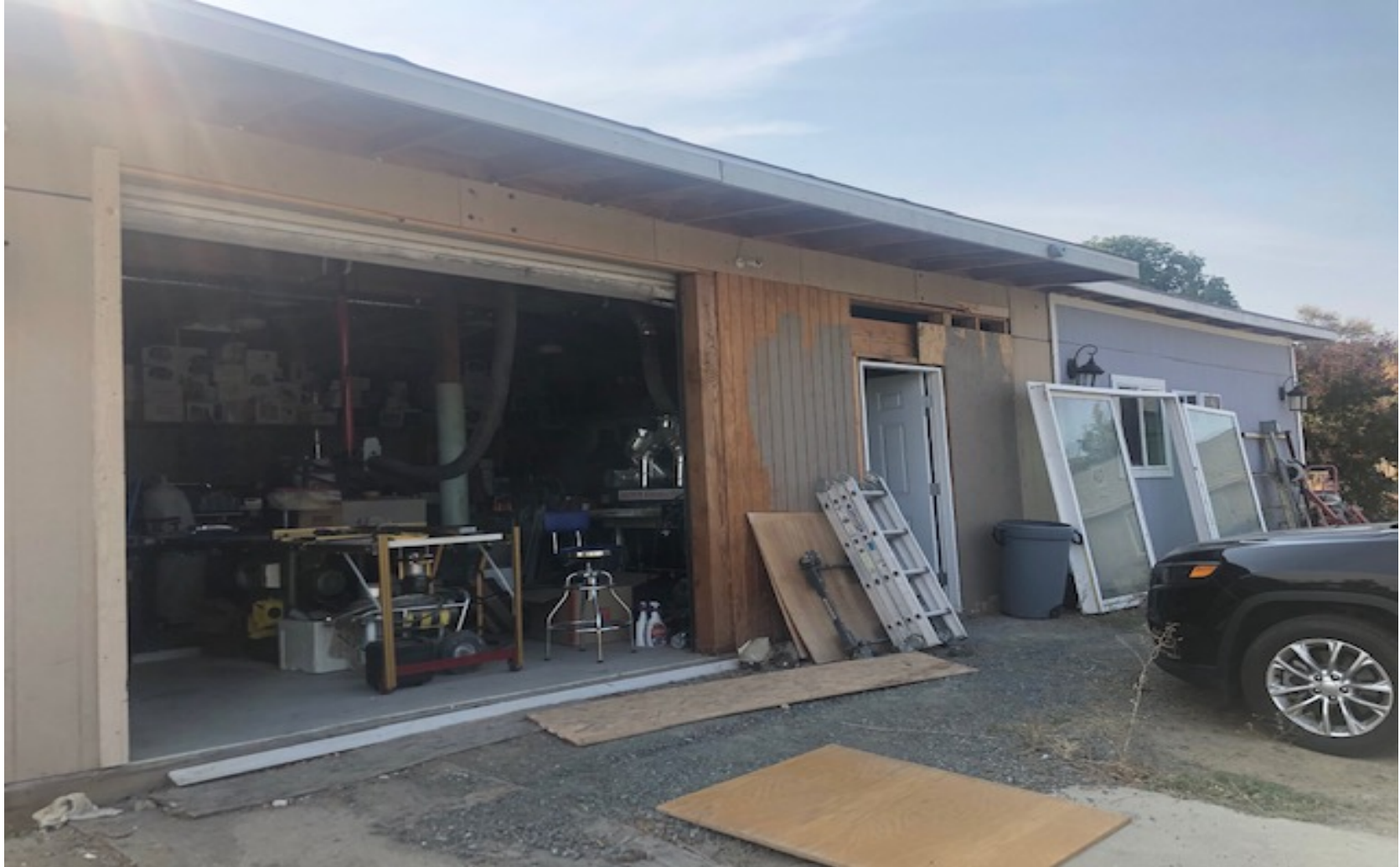
Workspace/Garage structure from the south
