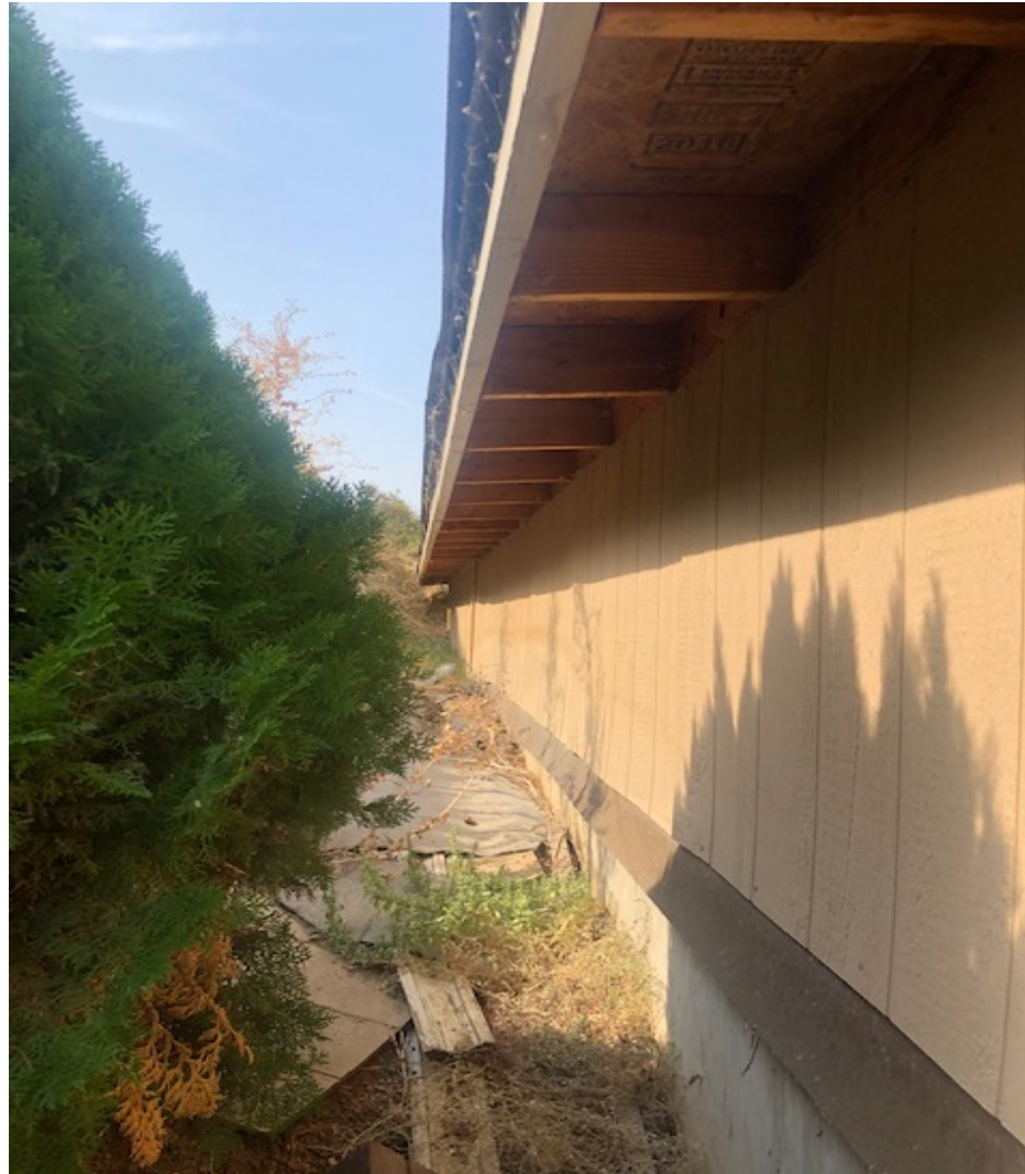
The northern elevation of the structure taken from northeast corner
