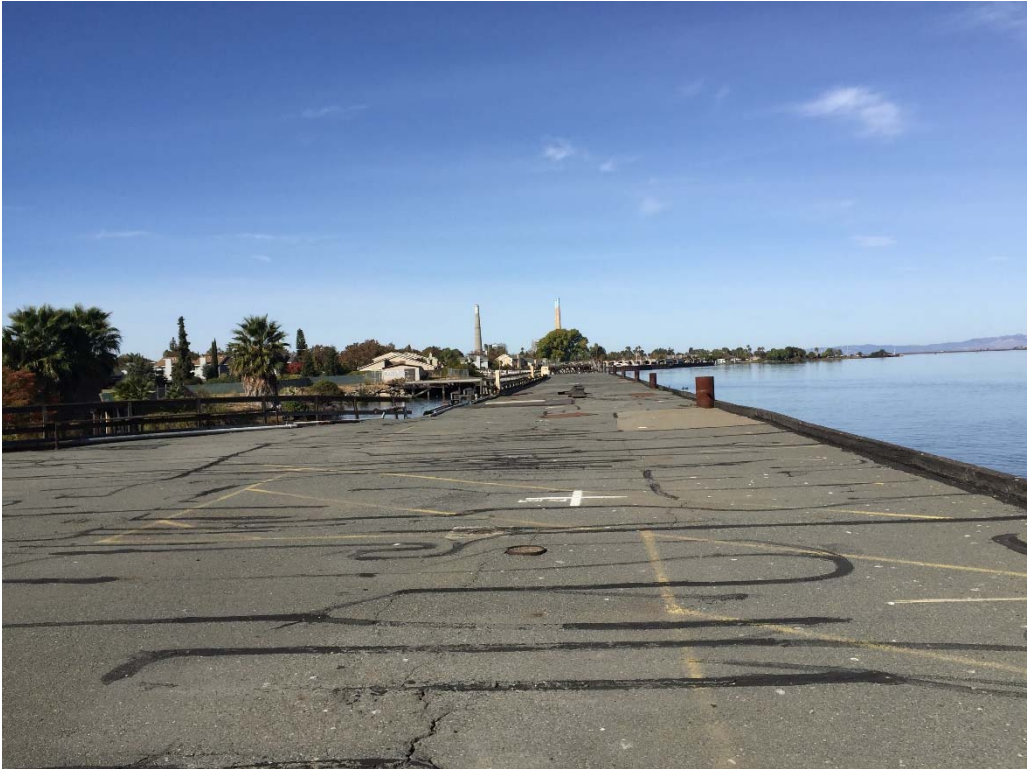
Terminal platform view
